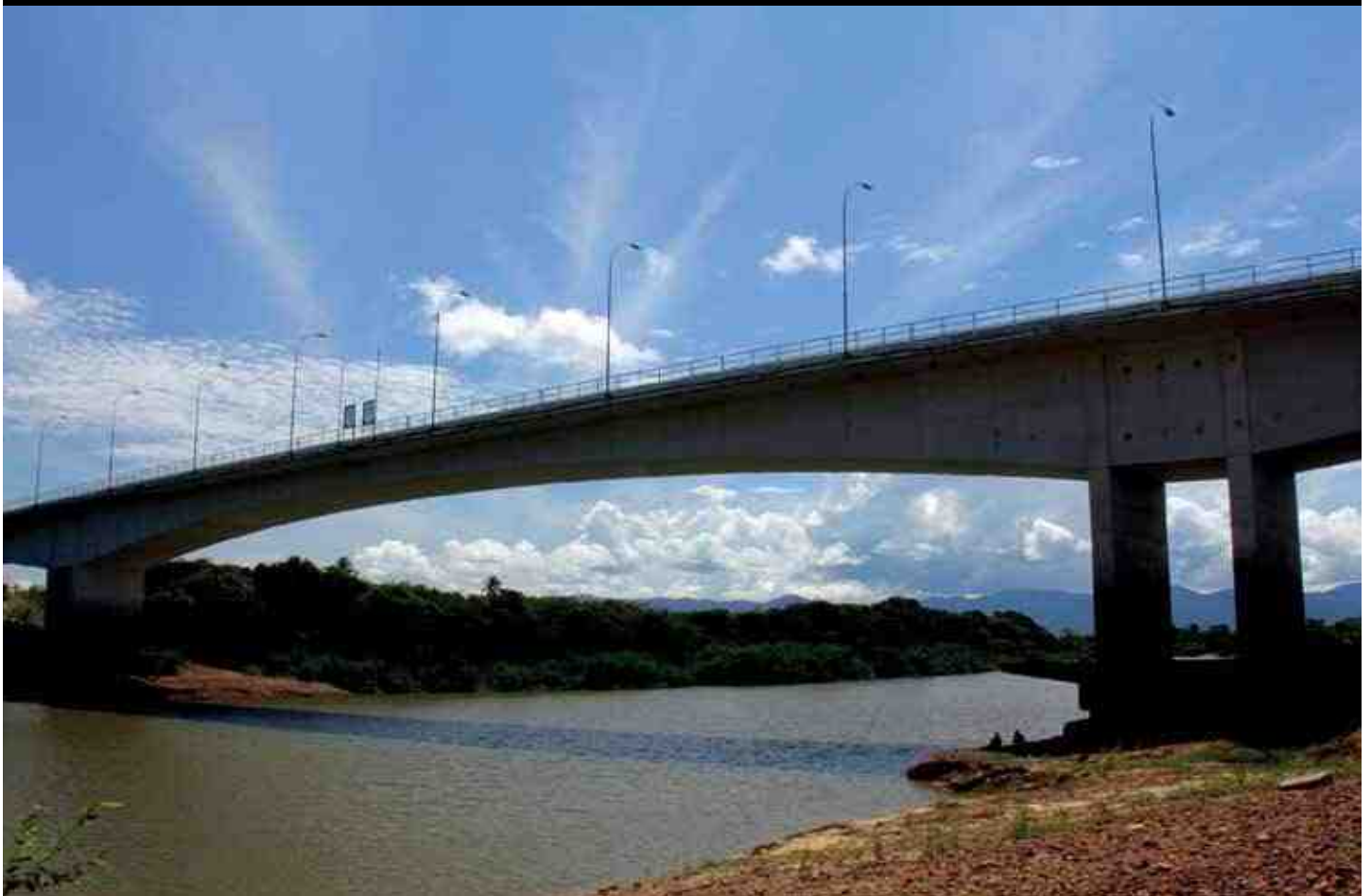
Ponte sobre o Rio Tacutu - Bonfim-Lethem - Bridge on the Tacutu River- Bonfim-Lethem
